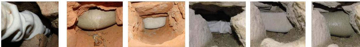
*Figure 1: Injection phases into brick masonry and stone masonry*
